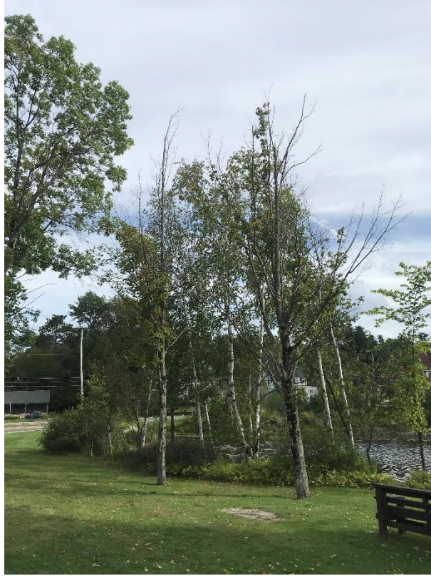
Figure 9: An example of a Priority 1 removal, dead tree near a bench.
